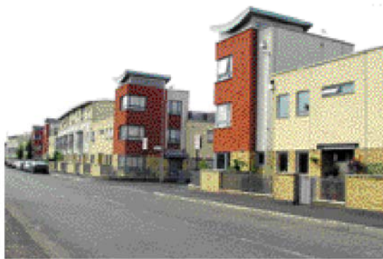
A mix of square and shallow plan dwellings provides a continuous street frontage. Rolls Crescent, Manchester
