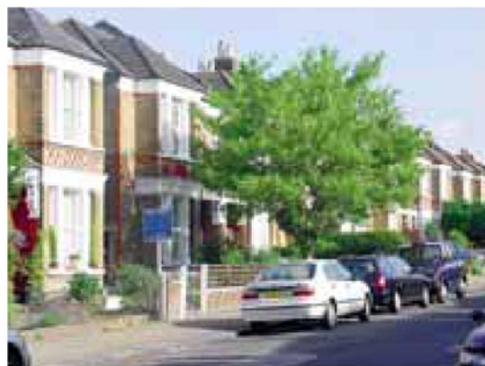
Narrow frontage, deep plan dwellings provide generous internal space and use land efficiently. Stanstead Road, Lewisham
